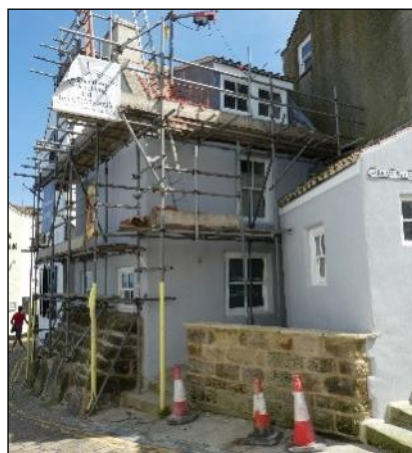
7. Sea Crest (YVBSG 1077) stands on a huge platform of natural rock, originally the base of a cliff, with the gable facing across the harbour. A lean-to kitchen belongs to the cottage but is structurally separate from it. Such 'detached kitchens' are a common feature of fishing villages on the North Yorkshire coast.
