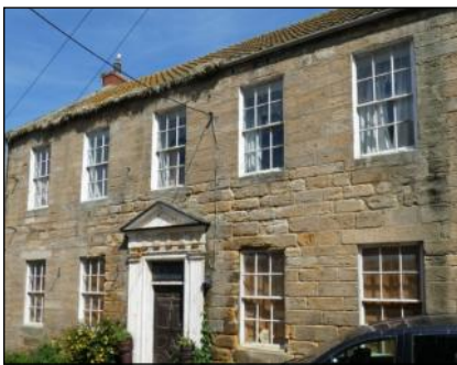
4. Kirkhill House (YVBSG 0925). Sadly, this house is now in need of some restoration. Likely built in the 1760s, the house was furnished with panelling, moulded door frames and a 'very fine' central staircase.
