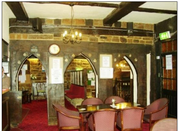
Right: the three doorways in an earlier partition at Baildon Hall
