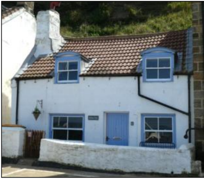
2. Harbour View (YVBSG 0933). This building is all that remains of a group of thatched cottages which were apparently arranged in a square. Storms washed away the other buildings. The outer wall was likely to have been built to protect the cottage from the scourge of the sea.
