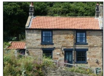
10. Numbers 4 and 5 Cowbar Bank (YVBSG 1941). A pair of cottages with a raised cruck between no 4 and no 5.
