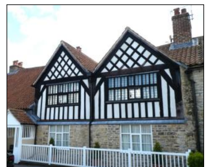
Old Manor House (YVBSG 0027). A timber-framed range, probably 17th century, presenting twin gables to the street, with a stone range to the left which has been used as farm buildings but was originally domestic.
