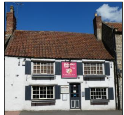
1 Bridge Street (YVBSG 0023). Central passage with main living room to left and smaller unheated room, the shop, to right. The building is similar to Thorpe's Cottage but it is not clear whether it has a timber frame.
