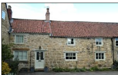
22 High Street (YVBSG 0100). Seems to have been designed as a traditional single-storey cruck farmhouse with cross passage. Later raised, rebuilt to left and extended at rear.
