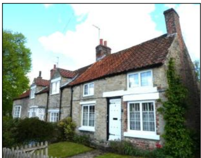
1 & 2 Buckingham Place (YVBSG 0025). Two adjoining and unequal houses, with an original core of a two-roomed house with later additions. Long range at rear.
