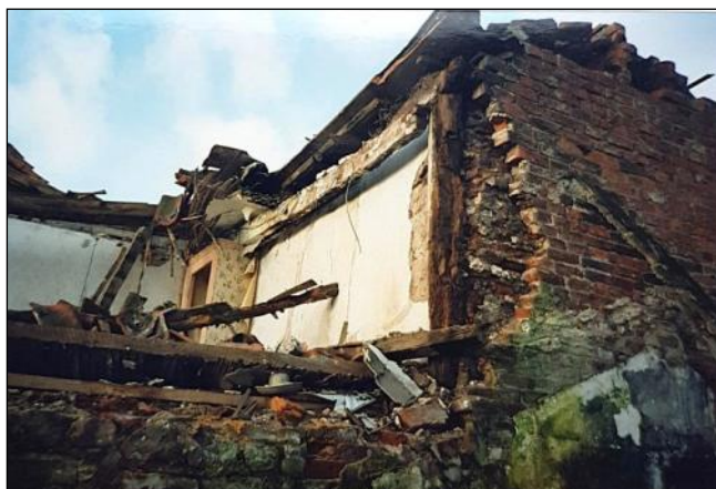
Demolished rear outshot showing timber framing
