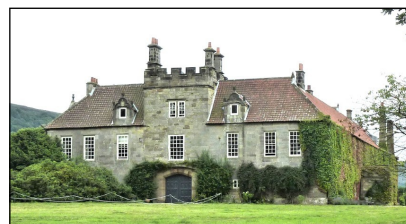
Ingleby Manor, Ingleby Greenhow (YVBSG 1860). A large double-courtyard house, probably of the mid 16th century. A mammoth recording task, undertaken over about eight years! See David Cook's article in Yorkshire Buildings No 46.
