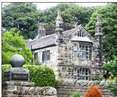
Fairfax Hall, Menston (YVBSG 1283). Originally a fairly small structure built early in the 17th century to serve a very specific purpose, possibly a banqueting house, as part of the more extensive Menston Hall.
