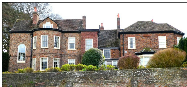
Fulford Hall, Fulford, York (YVBSG 0830). The brick manor house of Water Fulford dating from the 16th century with later additions and alterations, perhaps replacing a medieval house on the same site. Some roof timbers are re-used from timber wall-framing.
