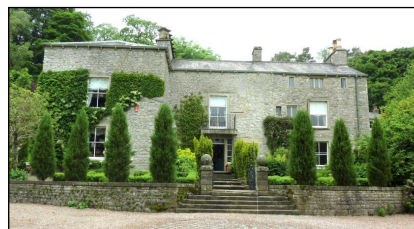
Austwick Hall (YVBSG 1740). Largely 16th century comprising hall and cross-wing, with linear service end rebuilt in the 17th century. Probably built on the site of an earlier manor house.
