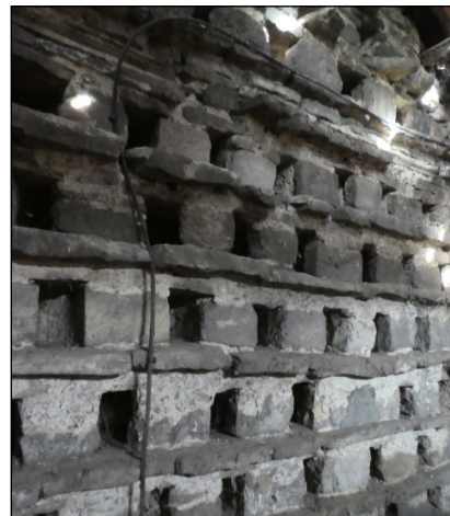
Norton Priory farm buildings, Norton, Doncaster (YVBSG 1913). A good collection of buildings including a hennery-piggery, stable and carriage house, granary barn, hay/threshing barn and horse engine house. The mid 18th century two-storey dovescote has about 340 L-shaped nest boxes on the upper floor. Outside is an alighting shelf below an opening which provides access for the birds.
