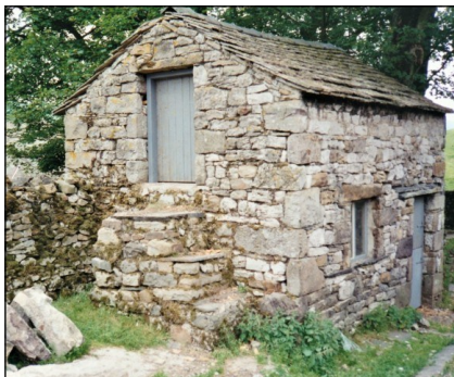
Hennery piggery at Low Birkwith Farm, Horton in Ribblesdale (YVBSG 1499). For housing hens above and pigs below, with the adjacent enclosure probably containing a feeding trough. The building was within easy reach of the farmhouse kitchen. Perhaps early 19th century.
