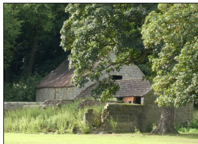
Pedigree bull mistal, Weston Hall, near Otley (YVBSG 1485). Probably late 18th or early 19th century, extended in about 1869 for the purpose of breeding pedigree bulls – single storey building raised to two storeys and bays added. Neaby in the same field are a set of dog kennels for otter hounds (YVBSG 1484), with space for food preparation, probably dating from the 19th century.
