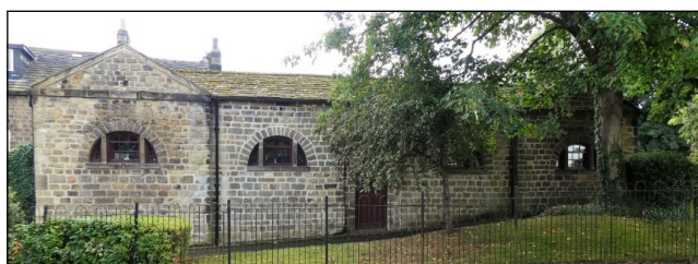
The Stables, Otley (YVBSG 1533). Part of Manor House outbuildings. Polite frontage of c1783 with evidence of older buildings including a possible single-storey cruck-built cottage. Used for a variety of agricultural purposes over the years.
