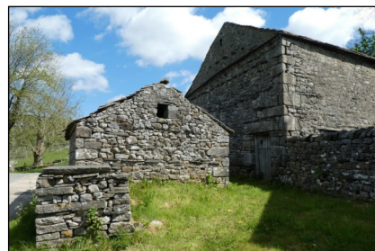
Outbuildings at Keepers Cottage, Brackenbottom (YVBSG 1489). A haybarn with integral shippin, and a separate midden house in front of it. Midden house has wide opening to take a cart to load manure to carry to fields. Barn probably 1730s, midden house a 19th century improvement.
