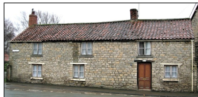
22 Ryegate (YVBSG 0109). Originally a single-storey cruck-framed hearth passage house. On the ground floor there are two parlours back and front, a housebody, the cross-passage and beyond it a dairy and scullery, perhaps formerly a cow-house or stable.
