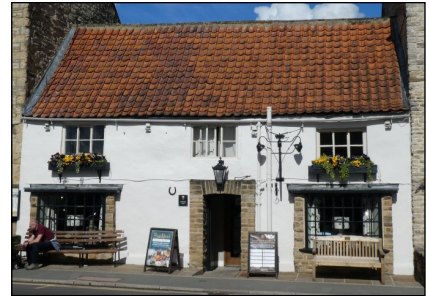
Thorpe's Cottage, 5 Market Place (YVBSG 0026). Built as a timber-framed house, probably of two storeys and three bays with central passage. The building is comparable with 1 Bridge Street.
