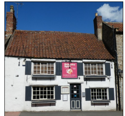
1 Bridge Street (YVBSG 0023). Central passage with main living room to left and smaller unheated room, the shop, to right. The building is similar to Thorpe's Cottage but it is not clear whether it has a timber frame.
