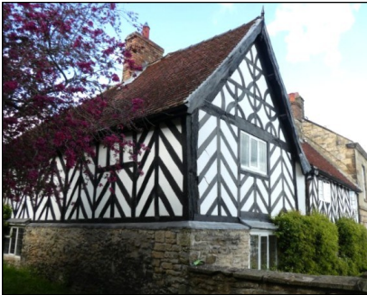
Rectory Manor House (YVBSG 0028). Hall and cross wing plan, separately framed. Service wing replaced by a Georgian house. Herringbone framing probably 16th century, style not local to this area.
