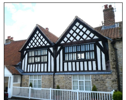
Old Manor House (YVBSG 0027). A timber-framed range, probably 17th century, presenting twin gables to the street, with a stone range to the left which has been used as farm buildings but was originally domestic.
