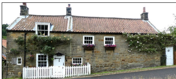
Old Lord Nelson, Beck Hole (YVBSG 0737). Originally a three-unit single-storey cross-passage house with thatched roof, built in 1678. Alehouse from at least late C18 to 1940. Cellar and bar parlour still there when recorded.
