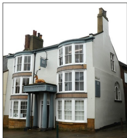
The Buck Inn, Guisborough (YVBSG 1786). An inn by the 1740s, and probably much earlier. Fine ashlar sandstone stonework of c1800, with top storey of brick. Interior mostly reconstructed about 1960 but remains of mud-and-stud partitions and a magnificent central roof-truss, probably c1600. Former maltings at rear.
