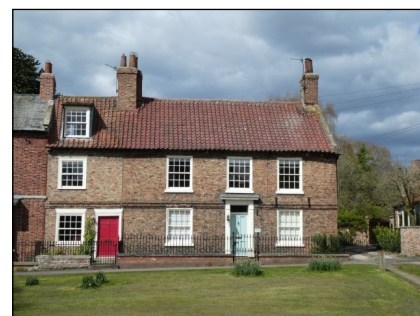
36 and 38 Uppleby (YVBSG 0782). Late 18th century house on the right, cottage added on the left perhaps c1840. The housekeeper for No 38 is thought to have lived in the cottage at some point. Re-used timbers in the roof, some with carpenters' marks relating to former uses.
