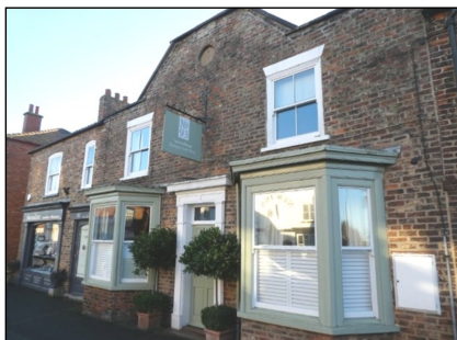
93 and 95 Long Street (YVBSG 0706). The house (No 93) appears to be purpose-built in the 19th century as a bakery, shop and dining room, with family living accommodation. The cottage (No 95) predates the house and is perhaps c1800 in origin.
