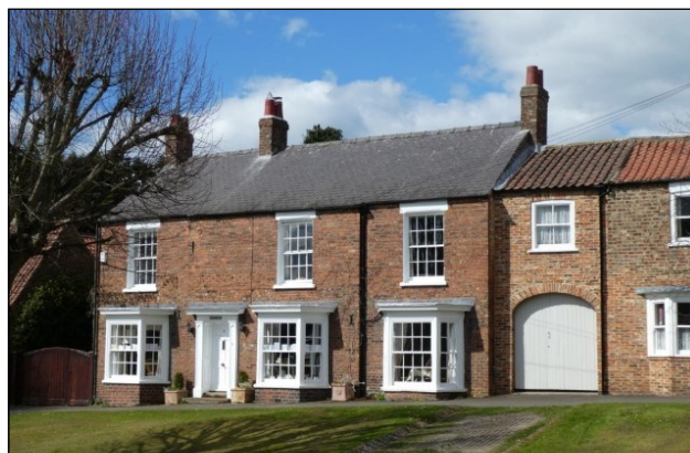
6 Uppleby (YVBSG 0762). Originally a timber-framed Vale of York type house with rear aisle, with walls rebuilt in brick in the late 18th century onwards. A wide-chamfered beam is stopped with 'Wern-hir' type stops, probably of c1600.
