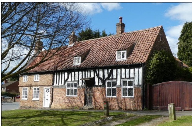
Tudor House and Cottage, Uppleby (YVBSG 0012). Formerly a single timber-framed 3½ bay house with ogee braces and rear and end aisles, probably of the 16th century. Contained two firehoods, one perhaps inserted later than the other.
