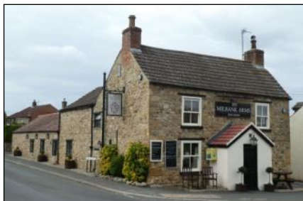
Milbank Arms, Well (YVBSG 0787). Used as an inn since 1882. Walling of cobble, with attached farm buildings also of cobble. Roof probably of cut-down full crucks re-used as raised cruck trusses with feet buried in stone walls, with one truss reconstructed a second time as an upper cruck truss with feet tenoned into a tie beam.
