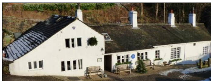
Bridge Inn, Ripponden (YVBSG 1297). Single-storey stone building containing one cruck truss, with two-storey wing at one end. Probably C16 to early C17, a more modest building than some timber-framed Calderdale houses.
