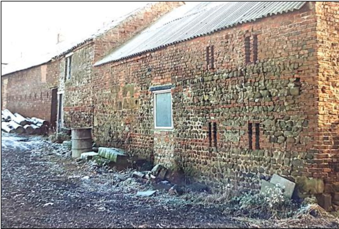
The range of farm buildings at Hillview Farm
