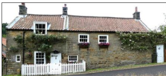
Old Lord Nelson, Beck Hole (YVBSG 0737). Originally a three-unit single-storey cross-passage house with thatched roof, built in 1678. Alehouse from at least late C18 to 1940. Cellar and bar parlour still there when recorded.
