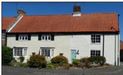
The Old Golden Lion, Topcliffe (YVBSG 0500). Perhaps mid C17. Mostly brick, with internal stud partitions. Flat staircase balusters may be connected with relocation of staircase and excavation of cellar when function changed from farmhouse to inn c1700.
