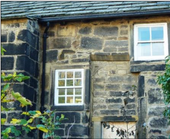
Altered openings in a wall at Calverley Old Hall
