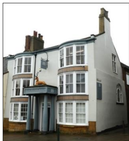
The Buck Inn, Guisborough (YVBSG 1786). An inn by the 1740s, and probably much earlier. Fine ashlar sandstone stonework of c1800, with top storey of brick. Interior mostly reconstructed about 1960 but remains of mud-and-stud partitions and a magnificent central roof-truss, probably c1600. Former maltings at rear.
