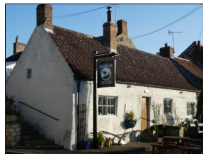
The Plough Inn, Wombledon (YVBSG 0329). Walling of limestone, with crucks which are crossed at the apex. Thatched until 1969. Thought to date from C17.
