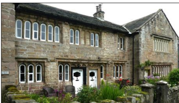
Left: round-headed mullioned windows at Roughlee Old Hall
