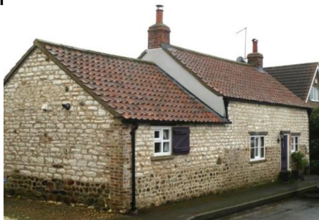
3 Pump Lane, Bempton. Chalk rubble cottage built on cobble foundations. The listed building description mentions a single roof truss with a tie beam which is a reused cruck blade, the two principal rafters possibly also being cruck blades.
