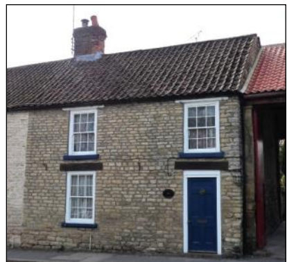
Roxby Farm Cottage (YVBSG 1766). Originally had gable facing the street. One cruck truss survives, with saddle dendro dated to 1574. Thick waney walls around the feet of crucks suggest an earlier stone plinth supporting earthen walls. Blocked fire window indicates later insertion of a firehood.
