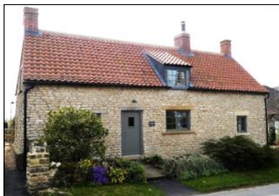
Woodbine Cottage (YVBSG 0888). Roof raised, formerly thatched. Cross-passage now stairs. Cruck blade re-used as purlin in bedroom.
