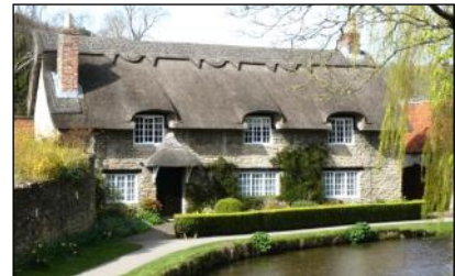
Beck Isle Cottage (YVBSG 0323). This picturesque much-photographed cruck-framed house was renovated 1938 when dormer windows were added and roof thatched with Norfolk reed. Contained a fine carved door to the C17 century spice cupboard or salt box.
