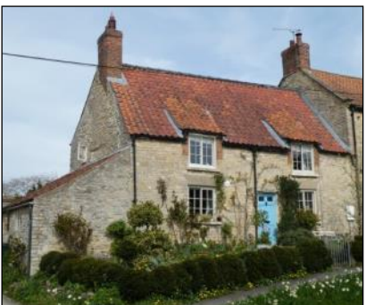
Westfield Cottage (YVBSG 1838). Roof originally thatched, unusually thick walls. Remarkably tall jointed cruck truss, certainly an original feature, not a repair as previously assumed. Cross-passage now integrated into neighbouring house.
