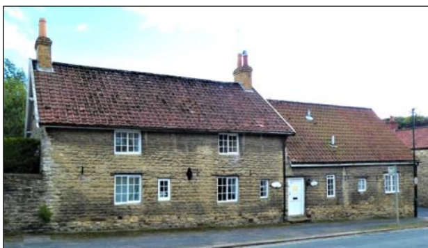
Church Farmhouse (YVBSG 0322). A former longhouse thought to date from C17. Contains two pairs of crucks. Date of 1704 on bressummer. Thatched until mid C20.
