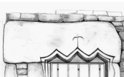
Hill Top Farm, Winewall, Trawden, near Colne – porch of 1661 has zig-zag lintel. Drawn July 2011.
