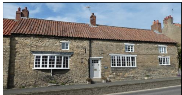
York House (YVBSG 0326). A four bay house which had crucks, cross-passage, speer, former salt-box and fire window at the time of recording. Wheat thatch was said to be covered by pantiles.
