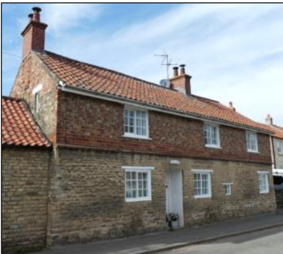
Walks View (YVBSG 0890). A 3-bay limestone cottage with first floor of brick. Contained one pair of crucks when recorded. Fire window survives but door to cross-passage now blocked. Thatched until early C20.
