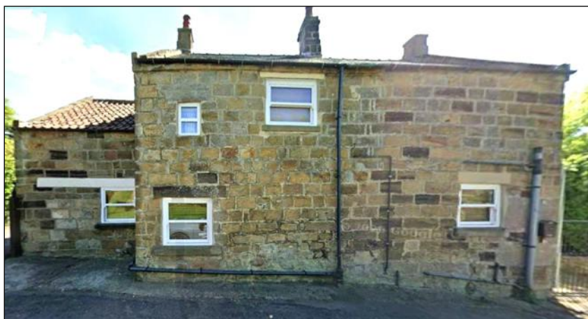
Rear of one of the stone cottages, Prospect Cottage in Micklehow Lane.
