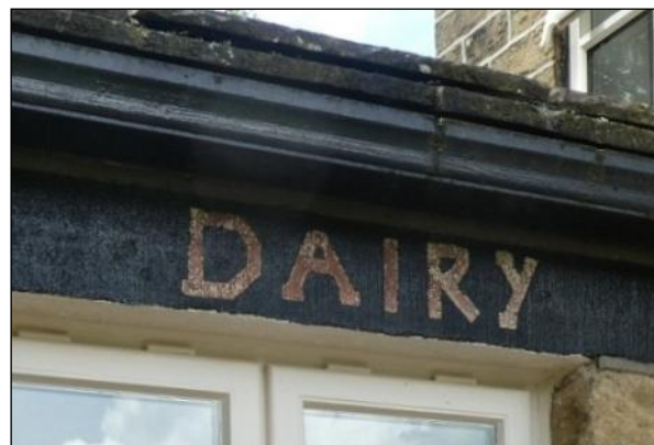
The dairy lintel at Rose Cottage, Brook Hill
