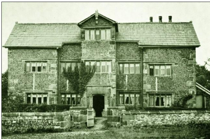
Carr House, photographed before 1955. The vertical channels between upper and lower windows are clearly visible.
