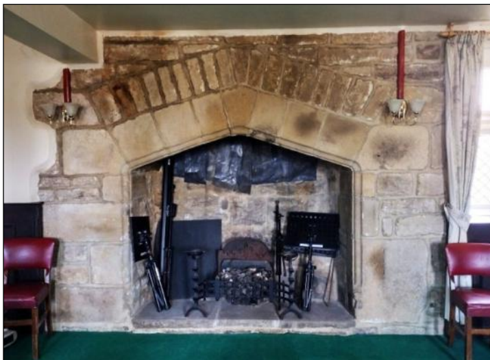
Baildon Hall: fireplace in chamber over hall
