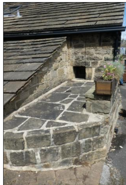
Cat flap and patio at Bank Walk House
