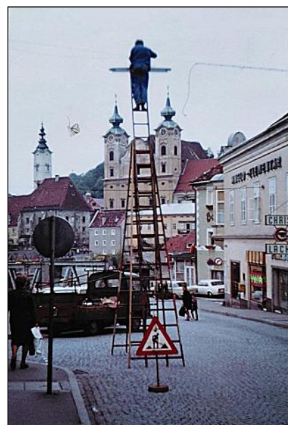
Interesting ladderwork at Steyr in Upper Austria 1971
