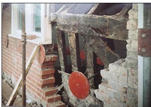
The timber framing revealed during works to No. 83 (Blacksmith's Arms), involving rebuilding of the dormers and parts of the front wall. Photographed 23 November 1988.
