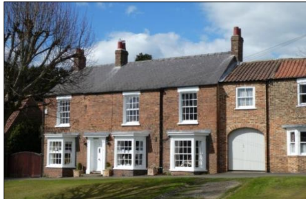
6 Uppleby (YVBSG 0762). Originally a timber-framed Vale of York type house with rear aisle, with walls rebuilt in brick in the late 18th century onwards. A wide-chamfered beam is stopped with 'Wern-hir' type stops, probably of c1600.
