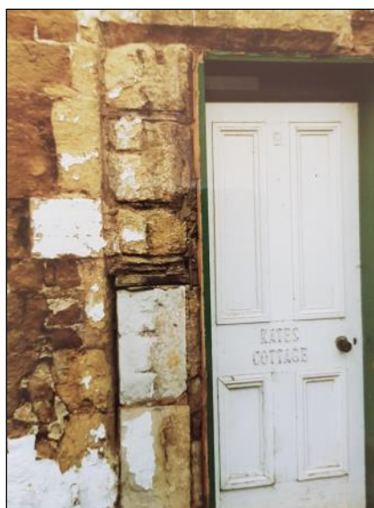
Older doorway revealed at Kates Cottage, photographed September 1989
