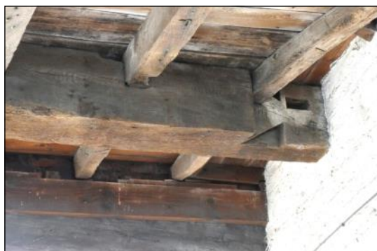
Re-used beam in carriage entrance
