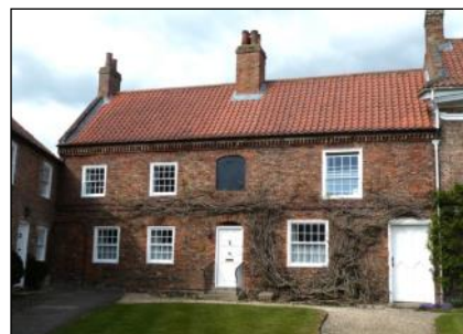
White House Cottage, Market Place (YVBSG 0769). Built 1700-1730 with re-used roof timbers which may be from an earlier house on the site. The adjoining house to the right, White House, has also recently been recorded by the YVBSG.
