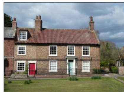
36 and 38 Uppleby (YVBSG 0782). Late 18th century house on the right, cottage added on the left perhaps c1840. The housekeeper for No 38 is thought to have lived in the cottage at some point. Re-used timbers in the roof, some with carpenters' marks relating to former uses.
