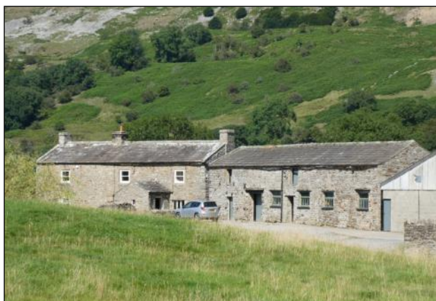
Town End Hall, Reeth, Swaledale (YVBSG 1248)
