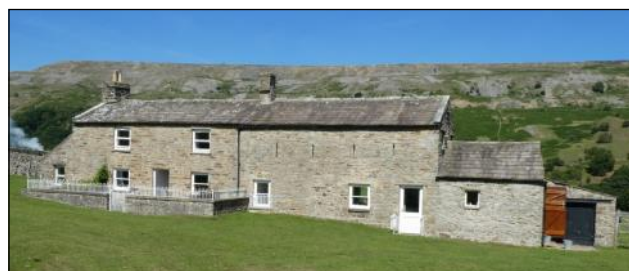
Lane House, Reeth, Swaledale (YVBSG 0440)
